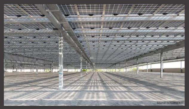
Roofing of multi-storey car park by integrated glass-glass solar modules
